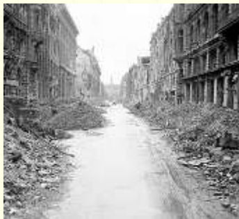
Bombed out street
